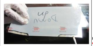
Draw conductive glue onto the cut. Make sure the conductive glue not touch the UNCUT smart glass film edges
